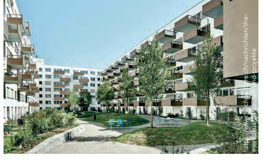
open yard situation Wohnüberbauung Sonnentalsstrasse, Zürich - ASP - shrubs to emphasise the private spaces - trees for intimacy - retentions moulds for seeping rainwater
